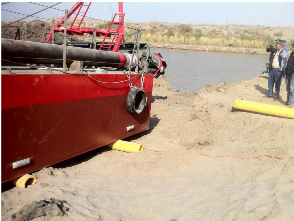
Figure 7 Preparing the “slipway”
