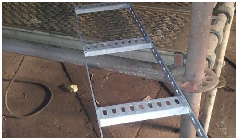
Figure 12 standard zinc-plated cable tray
