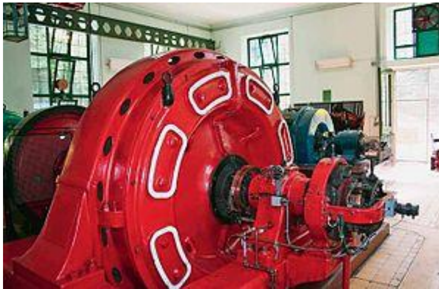
Slika 3.9 Peltonova turbina u HE Vinodol [11]
