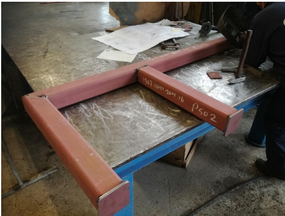
Slika 5 – Square tube foundation in production
