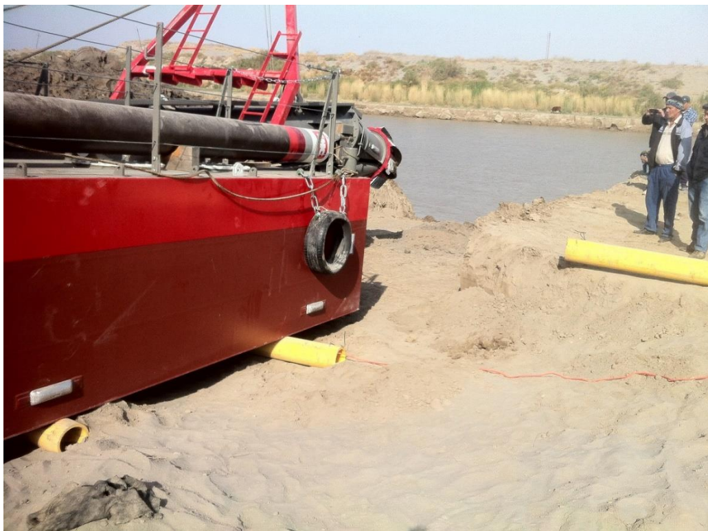
Figure 7 Preparing the “slipway”
