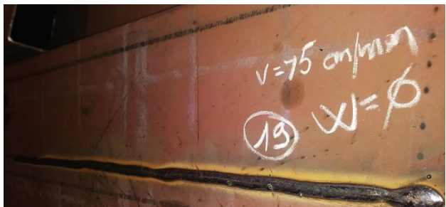
Figure 6 faulty tracking on weld no. 19
