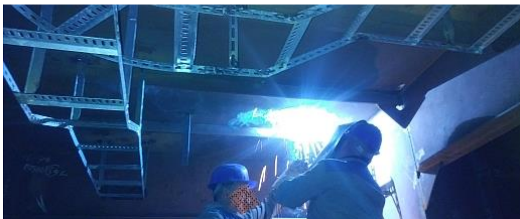
Figure 2 positioning and tack welding of cable tray
