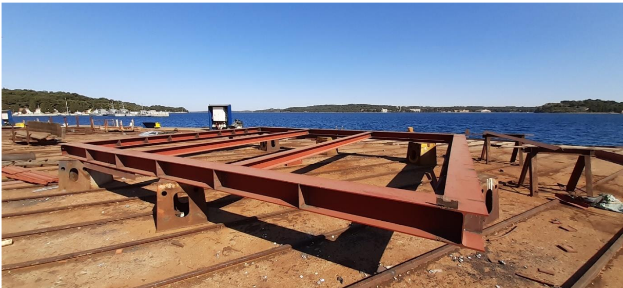
Figure 43 Demonstrator – steel structure under construction
