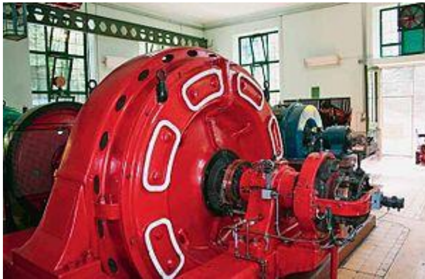
Slika 3.9 Peltonova turbina u HE Vinodol [11]
