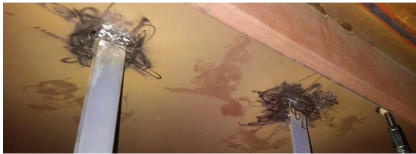
Figure 5 joint after welding and grinding. In right bottom corner stud weld could be seen which could give insight in difference between processes
